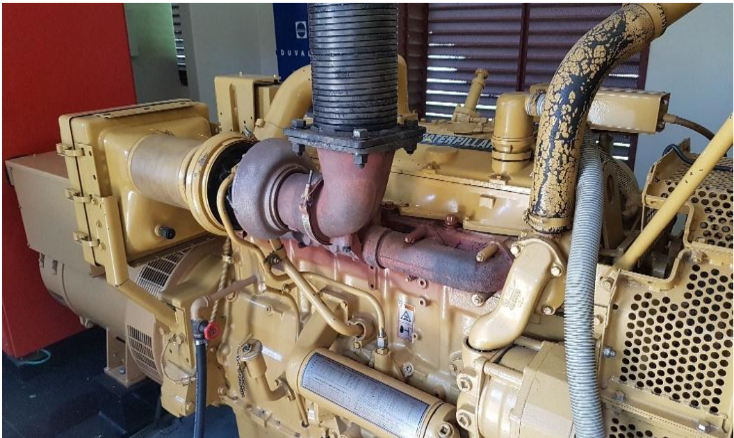
Figure 4-6: Diesel generator
