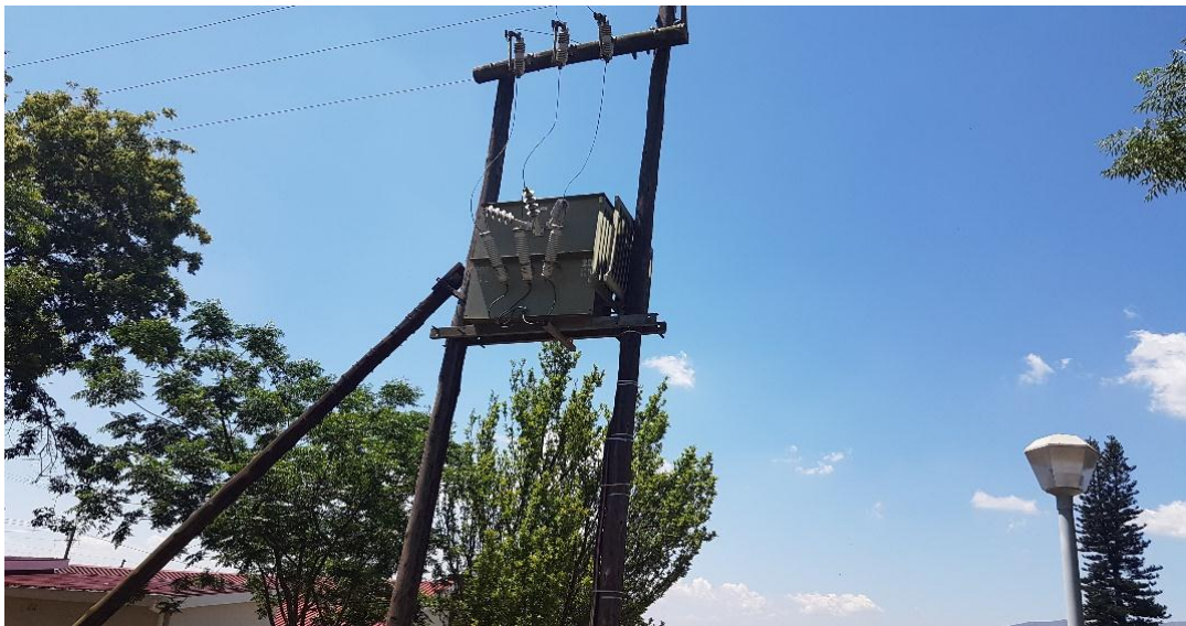
Figure 4-3: Pole mounted transformers located south of the main entrance
