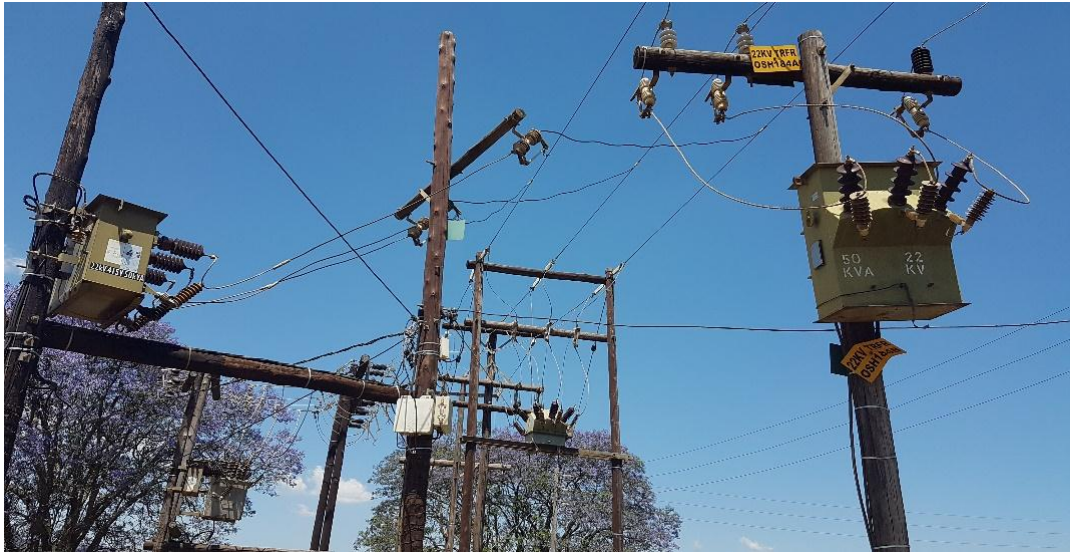
Figure 4-2: Two pole mounted transformers located directly to the right of the main entrance
