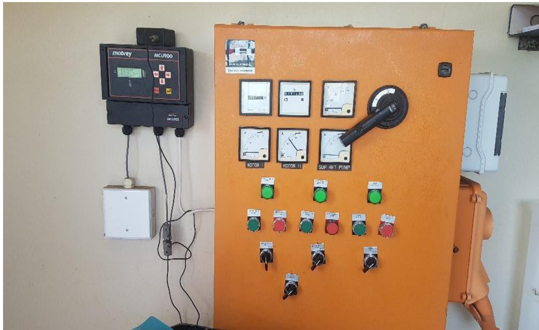
Figure 4-8: Rotor pump control panel for the waste water treatment plant
