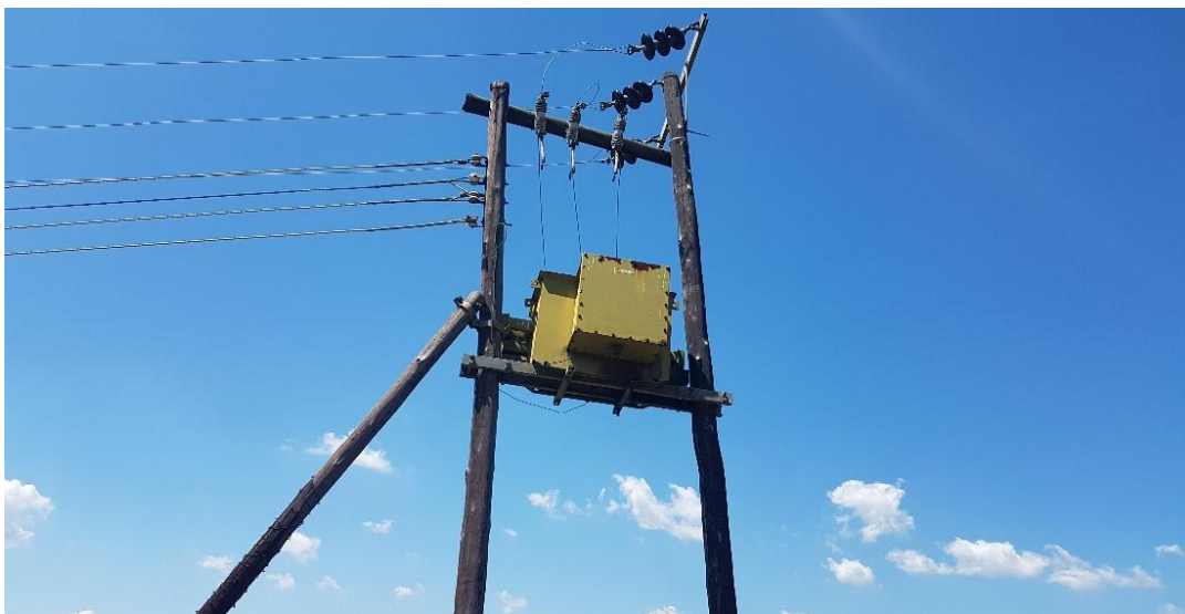
Figure 4-5: Disconnected pole mounted transformer located close to the water reservoir
